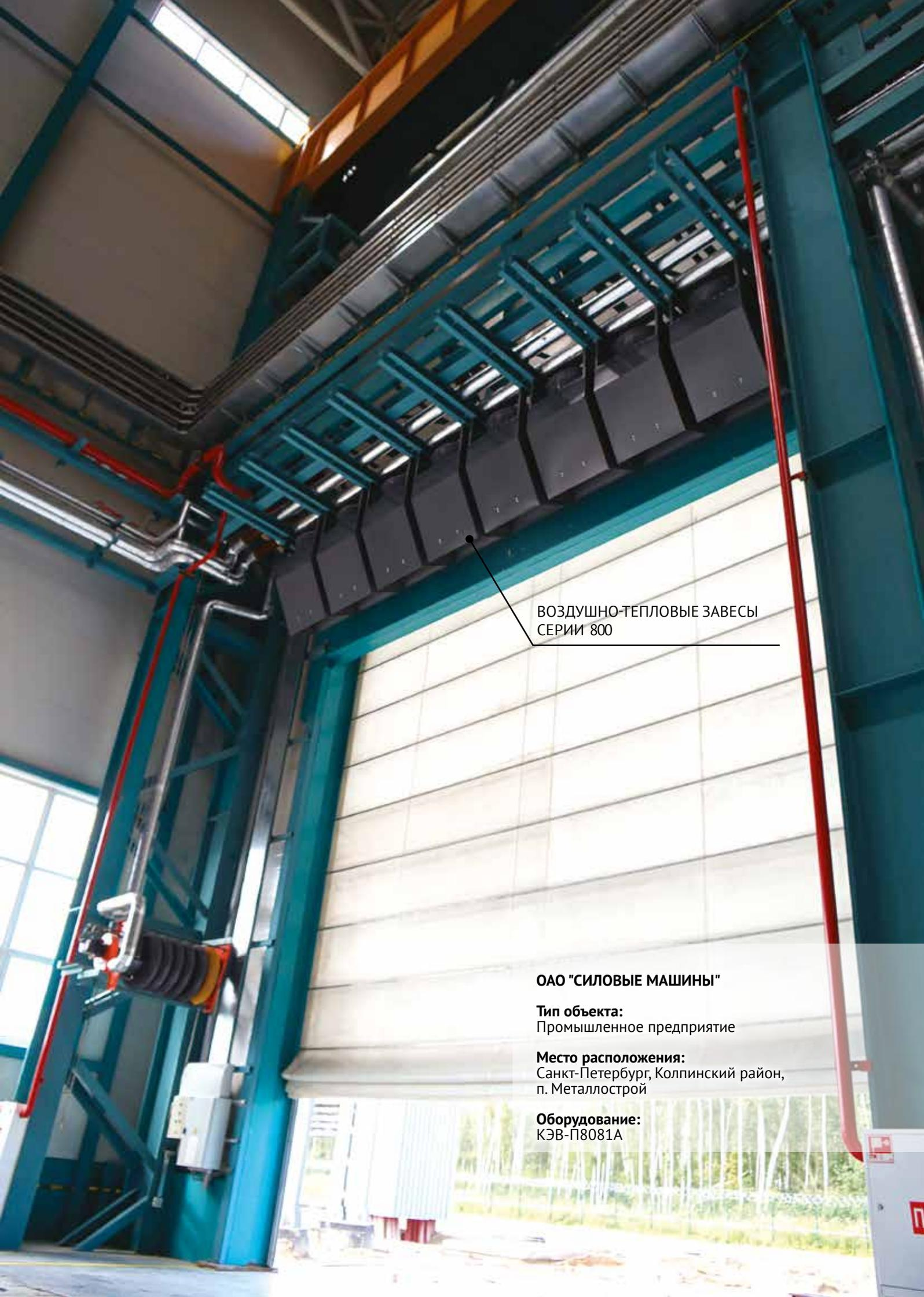
A photograph of an industrial facility, likely a power plant or manufacturing plant, featuring a large open bay door. The structure is made of blue-painted metal beams. Above the door, there is a series of air curtains (air curtains) made of dark, rectangular panels. The floor is concrete, and there are various pipes and electrical conduits visible. The background shows a bright outdoor area with trees and a fence.
